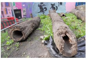
Elm was a popular choice for water pipes as, unlike other woods, it does not decay when kept permanently wet. Logs were bored lengthwise and tapered at one end to fit snuggly into the next length of timber. If each elm trunk was 4 meters long, it would take 2,000 elm trees to give enough pipes to run the 8 km from Swanston to Castlehill.
