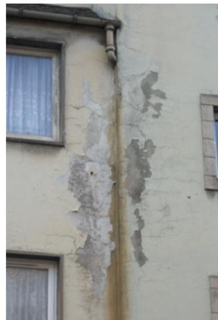
*Fig 6: flaking masonry paint*
