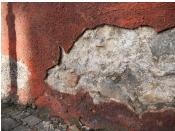
*Fig 4: detached cement render on lime-built wall*
