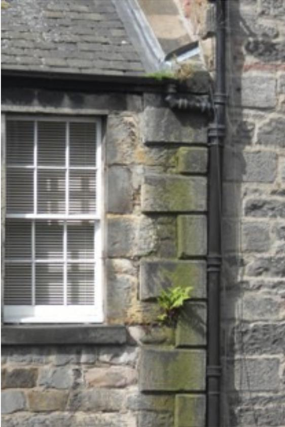
*Fig 2: blocked downpipe*
