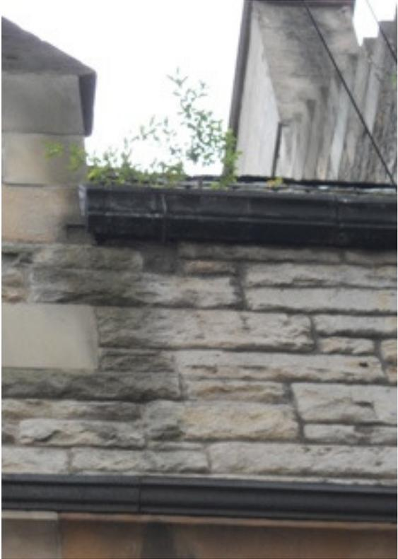
*Fig 1: tree in gutter*
